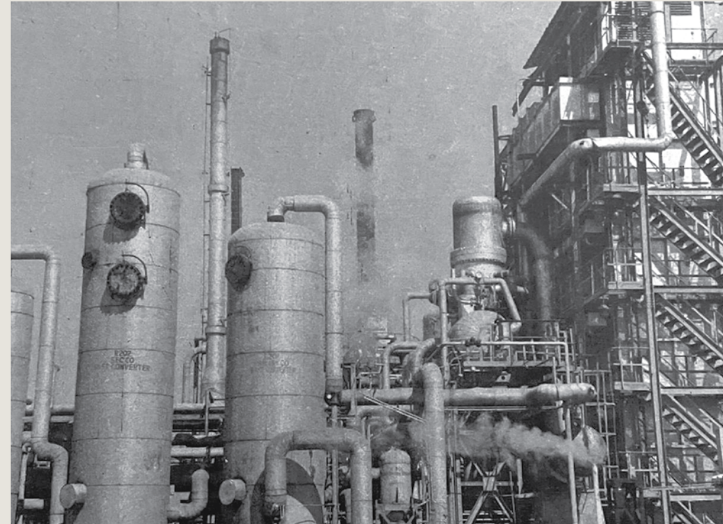
120 TPD Ammonia Plant at Udyogamandal
