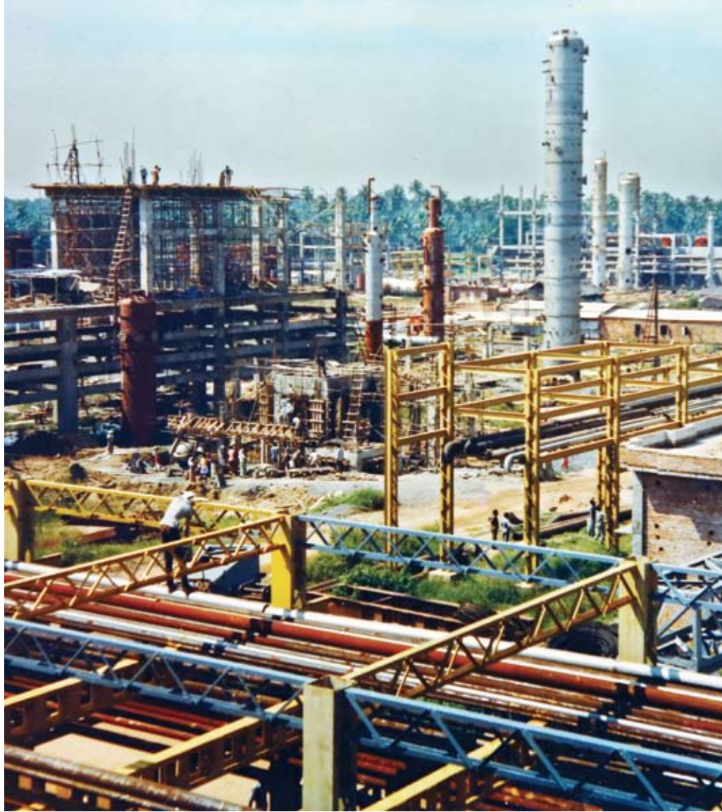
Construction of Lactam Plant in progress (old pic)
