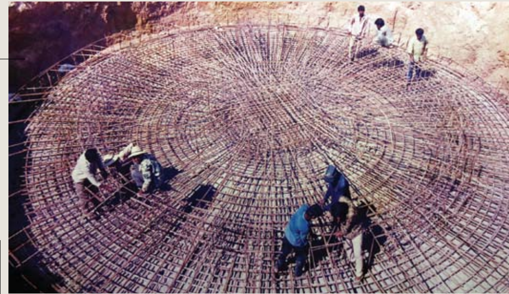
900 TPA Ammonia Plant Construction in progress
