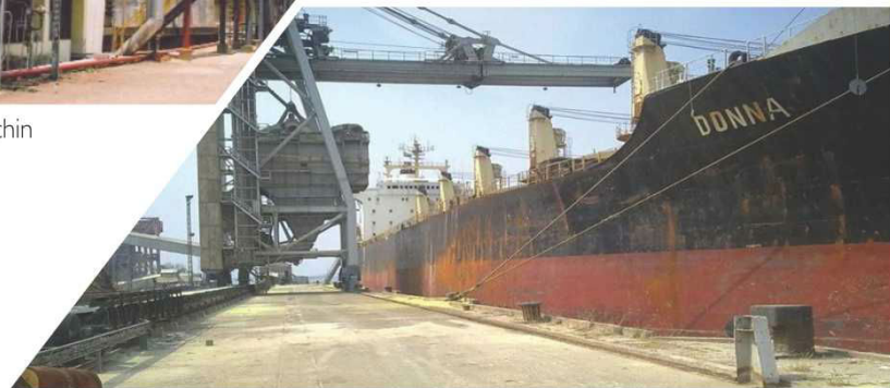
Hindalco – Ship unloading facility, Dahej
