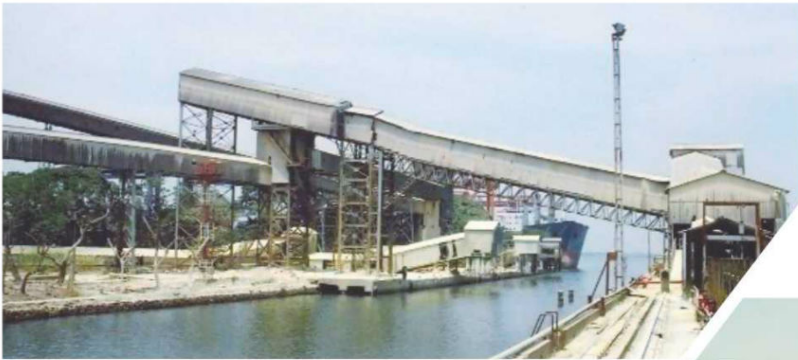
Rock phosphate/Sulfur handling system, FACT Willingdon Island, Cochin
